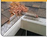
Roof valleys can cause excessive rain water and debris build up creating challenges for all gutter guards. Rainwater diverters help hold debris back and away from the gutter guard.
